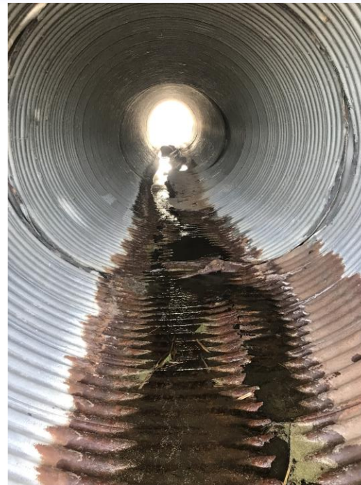
Culvert installed in the early 1980s
